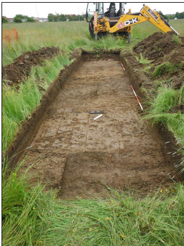
Figure 5. Trench 2 looking south east. Scales = 2 x 2m.
